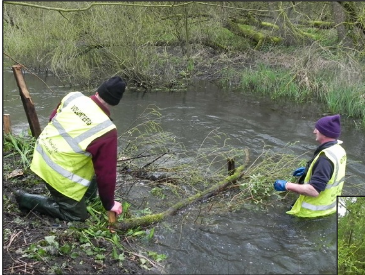
Bruce and Dick building a deflector. [Sue Frearson]
